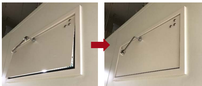
Energy saving by effective control of differential damper (Engineering & development center)
