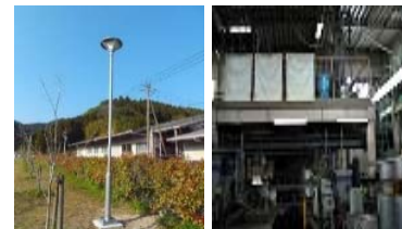
LED lighting (MIYAZAKI FUJITSU COMPONENTS)
