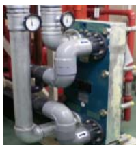
Exhaust heat is re-used for water heating (Engineering & Development Center)
