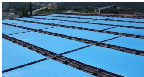
Shinano Fujitsu Limited Heat shield sheets on factory roof
