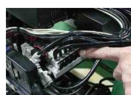
Energy saving by treatment against air leakage
