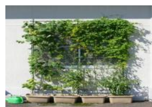
Heat rejection by Green Curtain Miyazaki Fujitsu Components Limited
