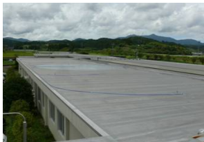
Improvement of air conditioner efficiency by watering on roof
